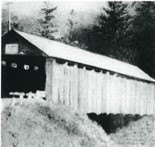
Blair Rd Covered Bridge 150 feet long Perry Township 1860- 1951
